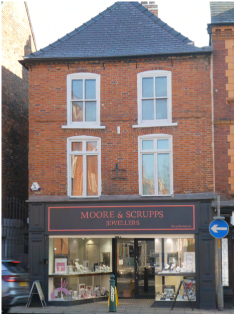
3, Southgate - Moore & Scrupps. A beautiful full face-lift from ground floor to chimney stack
