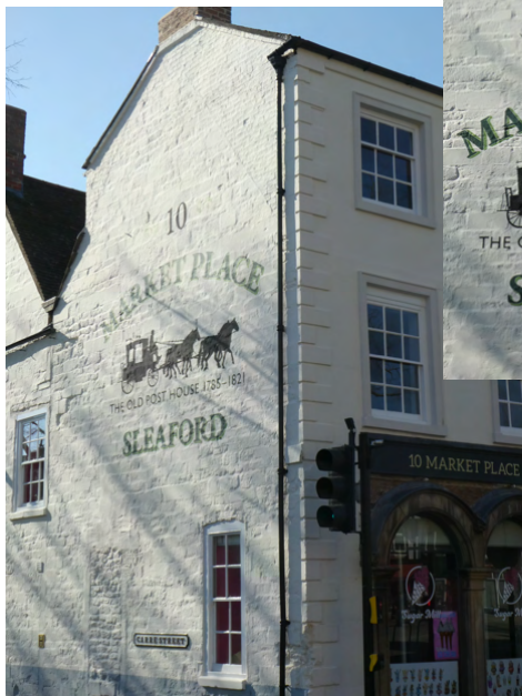
10, Market Place This Grade II listed building, the remains of one of the town's main coaching inns, now proudly displays it's heritage!
